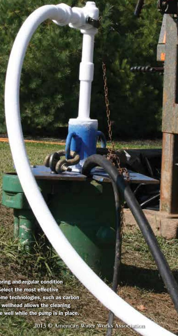
Effective well performance monitoring and regular condition assessments allow personnel to select the most effective rehabilitation technology. With some technologies, such as carbon dioxide, hardware installed at the wellhead allows the cleaning technology to be installed into the well while the pump is in place.
